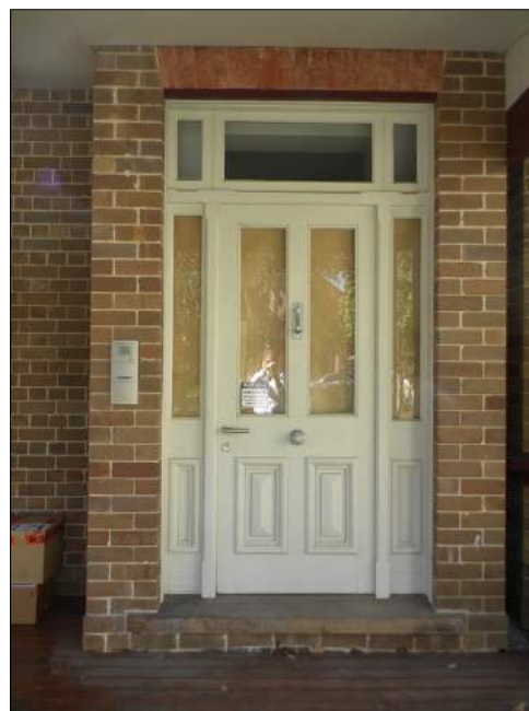
Figure 25: Detail of the front door. Note how the verandah lining partially concealed the brick headers above the door.
