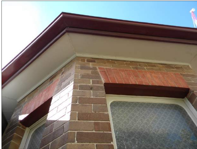
Figure 19: Modern square guttering and enclosed eaves.
