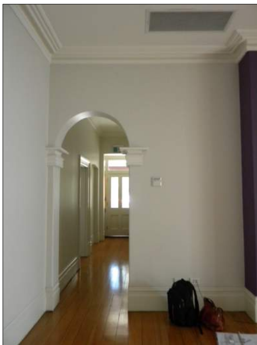
Figure 25: The arched entrance into the hallway from Room 4. The plaster capital detailing is replacement fabric.
