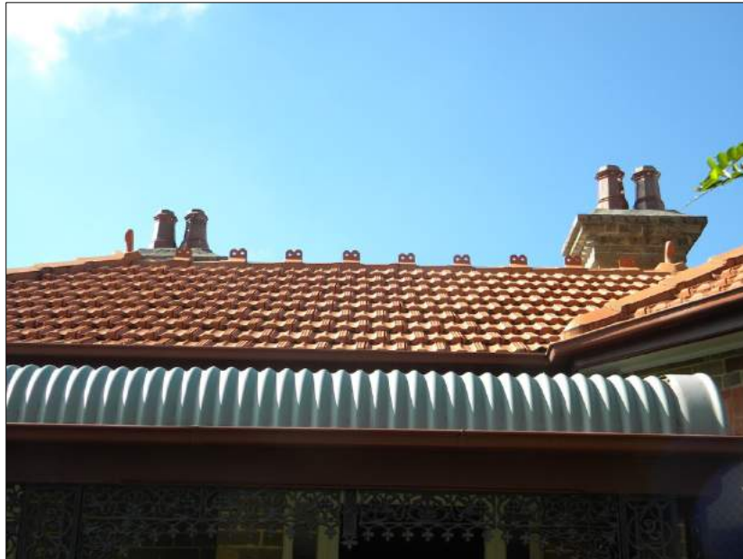
Figure 17: Terracotta roof and decorative ridge capping.
