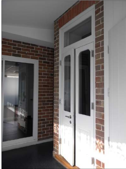
Figure 30: French doors set within a projecting bay. Figure 31: Timber threshold and detail of the bolection moulding.
