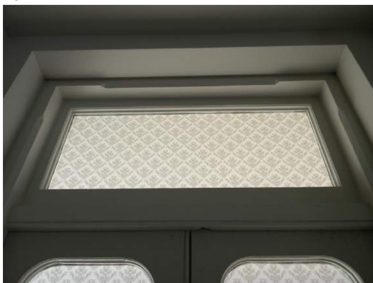
Figure 17: Detail of the architraves of the french door.
